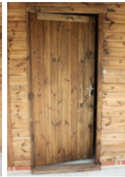
Joinery class door with keyed lock
