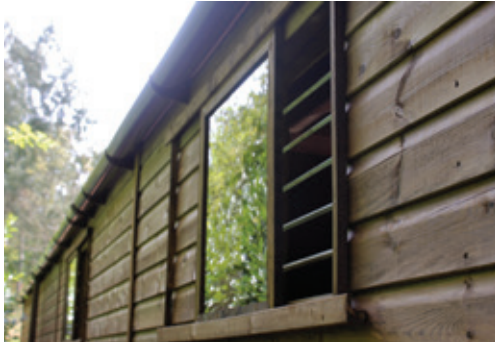
Rear (or front) sliding window with grill
