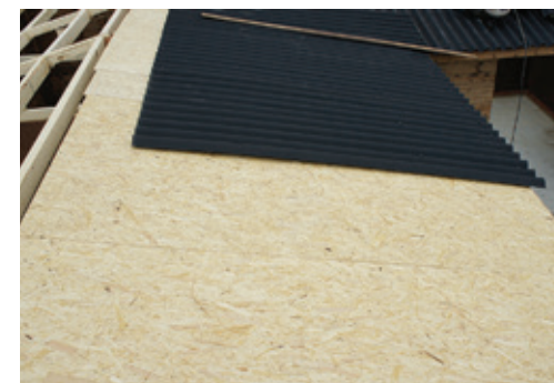
Roof decking supporting onduline to give a far superior, trouble free life - recommended
