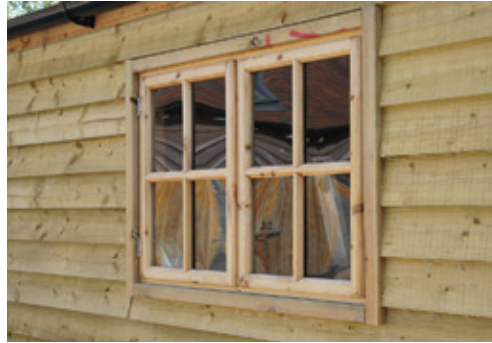
Cottage window with perspex infill
