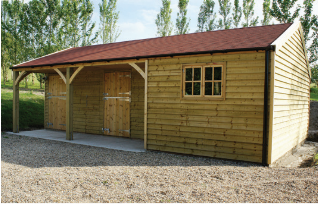
Felt tiles and rustic looking weatherboard cladding offering animal housing or storage and an adjoining office in the Ashdown Forest.
